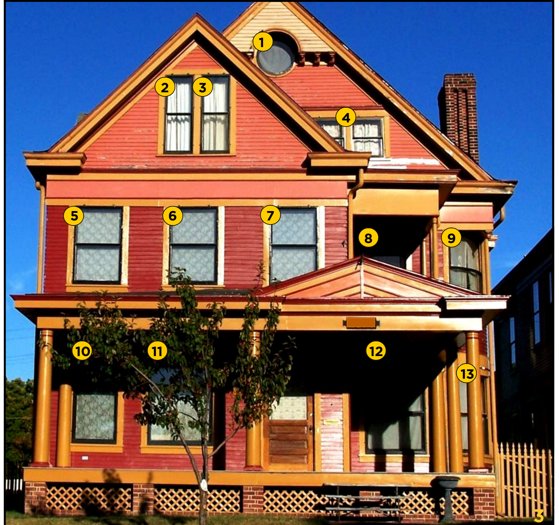
1890s Queen Anne style house Original one-over-one double-hung sash windows with storm windows
