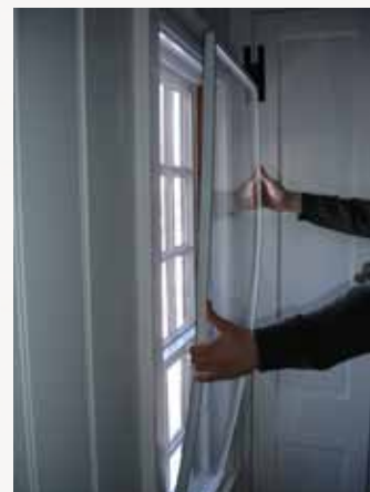
Interior storm panel.
